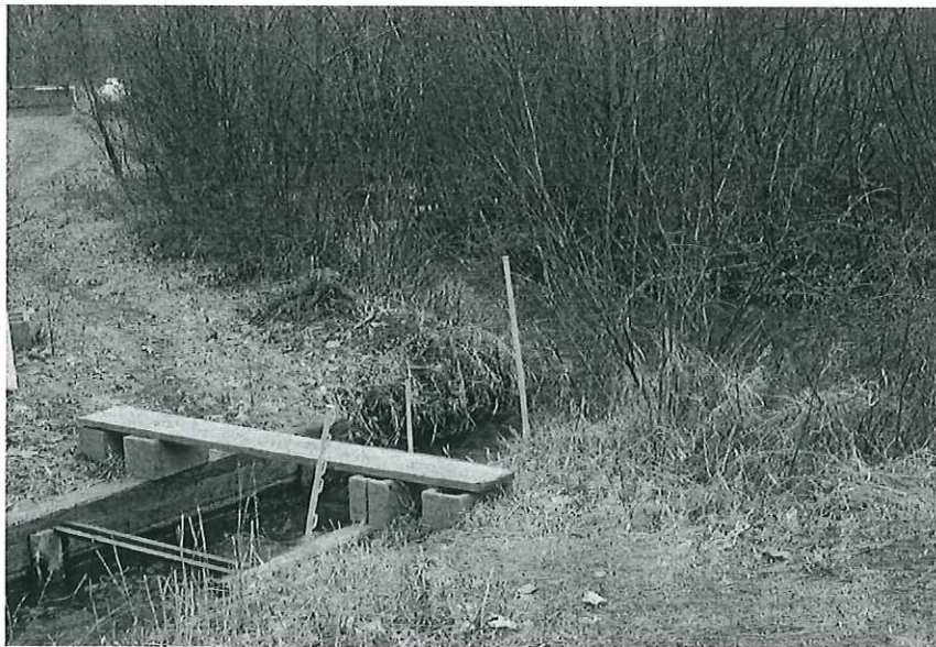
New, temporary gate in ditch for side channel diversion, created by Inouye in 2010
