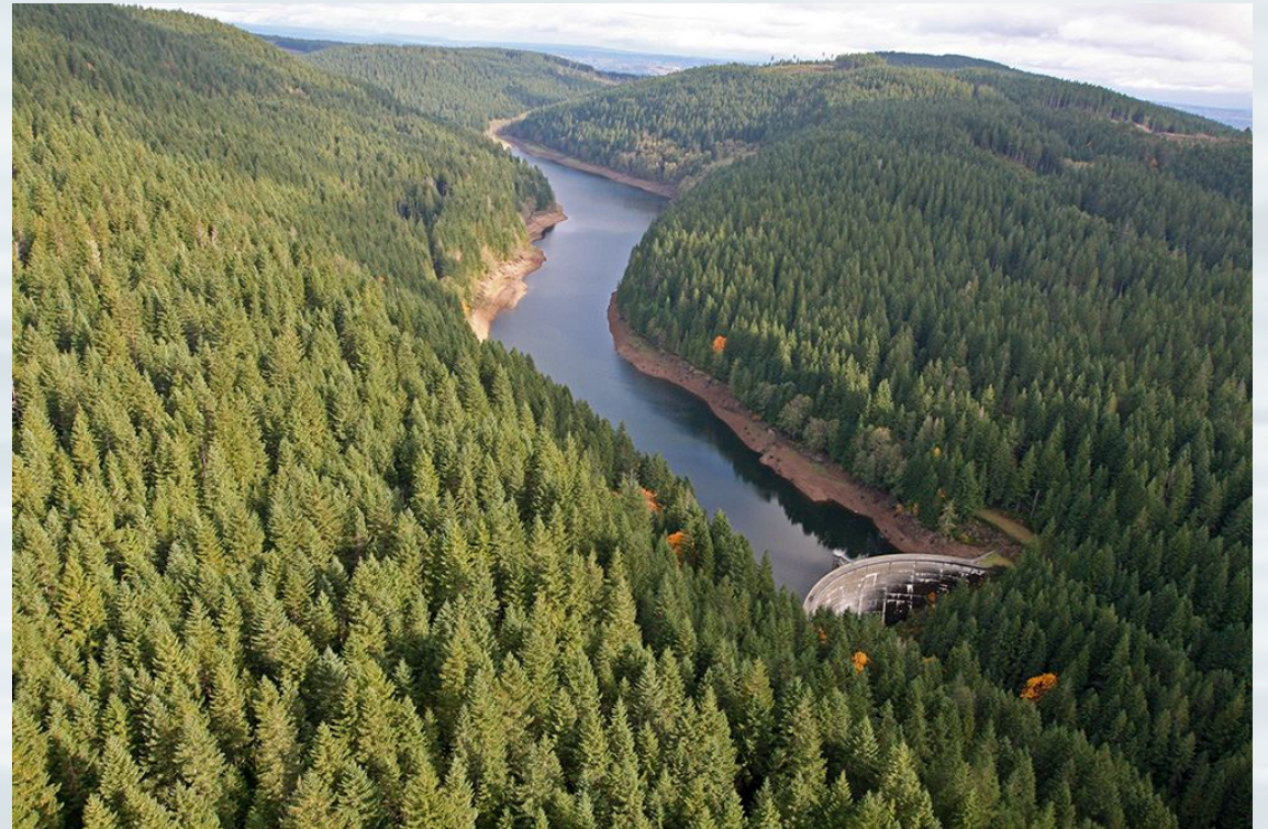
Casad Dam, Bremertonwa.gov
