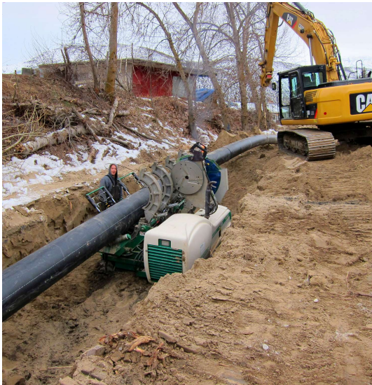
Lower Wenatchee in-stream flow enhancement project
