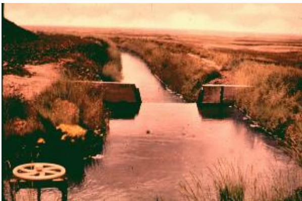
Figure 8. Condition of water approaching the weir is good, length of straight flow good, surface smooth and flow is slow
