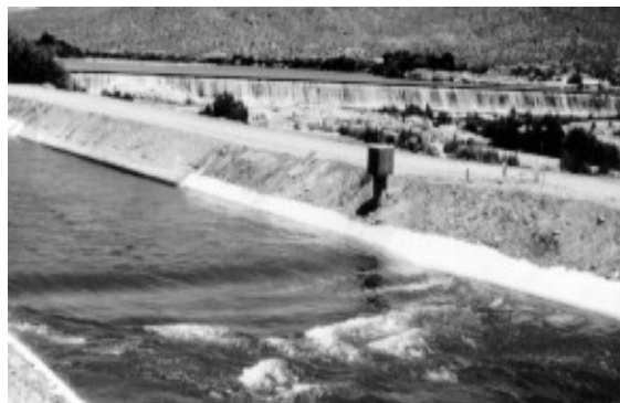
Figure 15. Long-throated ramp flume showing construction and operation in a large diversion canal
