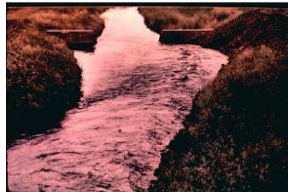
Figure 9. Conditions of water approaching the weir are incorrect, flow is not straight, surface is rough and flow is too fast
