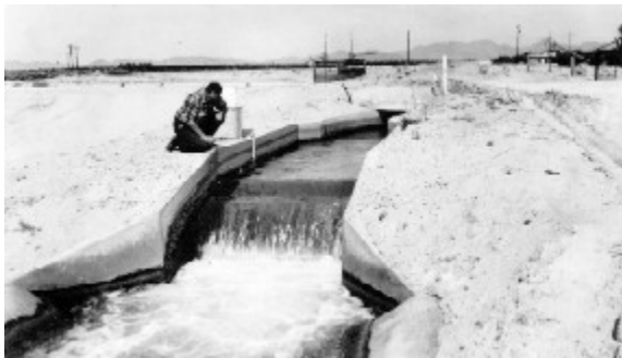
Figure 6. Example of a suppressed rectangular weir.
