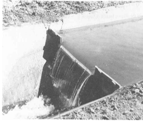
Figure 5. Example of fully-contracted rectangular weirs (note that h_o is the head (or depth) of the water flowing over the weir). This type of rectangular weir requires a weir blade with sides.
