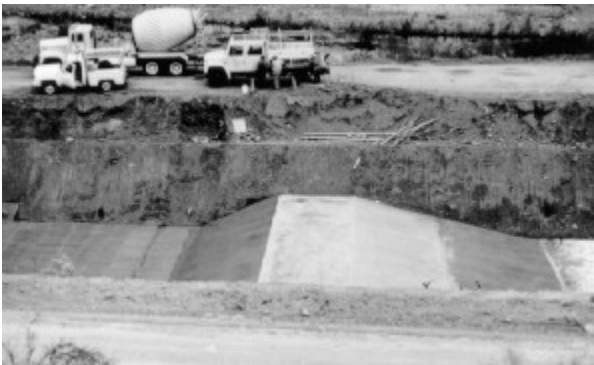
Figure 15. Long-throated ramp flume showing construction and operation in a large diversion canal
